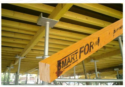
SmartForm is a Laminated Veneer Lumber (LVL) Engineered Wood Product used in concrete formwork support structures such as joists, bearers, walers and soldiers in conventional soffit formwork and vertical forms for concrete slab pouring.
